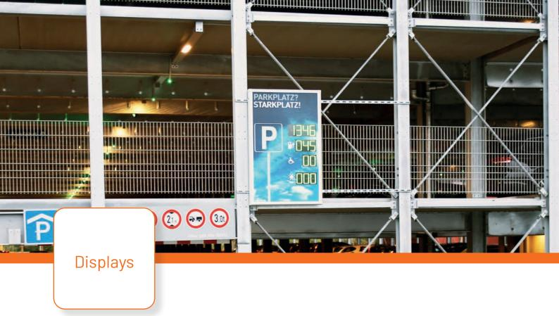
The first impression is what counts! A free choice in the design of the displays makes almost everything possible. Installation is possible on the mast or on the parking lot facade. The display has a series of green and red LEDs to display numerical information about the parking lot occupancy.
