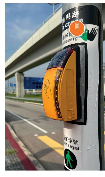
push button functions can be controlled via the network, while only two wires are required for the power supply. The two LED light modules are dimmable and can be operated at reduced luminosities in the dark.
